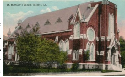
Historic postcard of St. Matthew's Catholic Church, built ca. 1890. Photo from http://www.alexandria-louisiana.com/monroe-louisiana.htm
