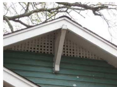
Trim such as eave brackets should not be removed or concealed (1015 N. 5th Street).
