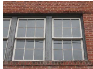
Six-over-six wood sash windows at 117-121 Hall Street.
