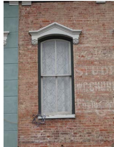
Original two-over-two wood sash window with ornamental hood at 120 S. Grand Street.
