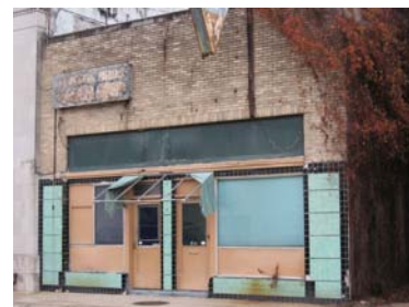
The transom at 103-105 Catalpa Street could be uncovered as part the of building's restoration.
