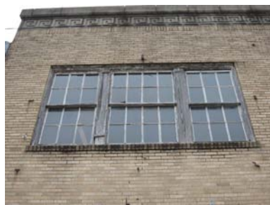
Original six-over-six and eight-over-eight wood windows at 404-408 Desiard Street. This window is significant to the design and character of the building.
