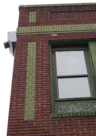
Textured and tinted brick adds much of the character to this commercial building at 111 Catalpa Street.
