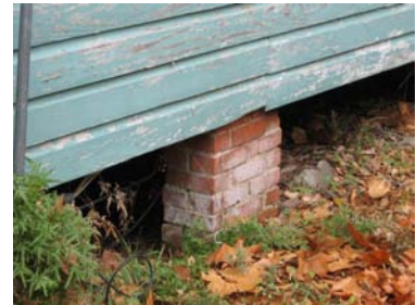
Brick pier foundation at 1015 N. 5th Street.
