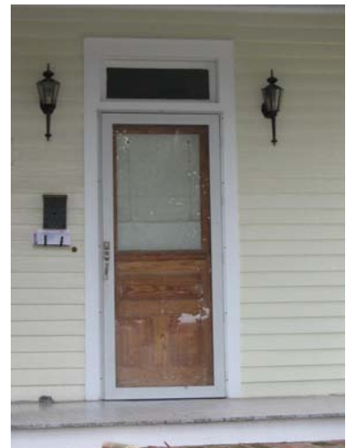
An appropriate storm door at 400 McKinley Street does not conceal the original wood door behind it.
