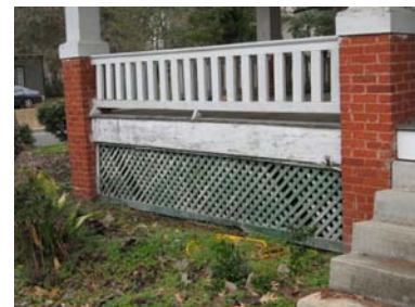
Lattice is an appropriate addition between piers (1001 St John Drive).
