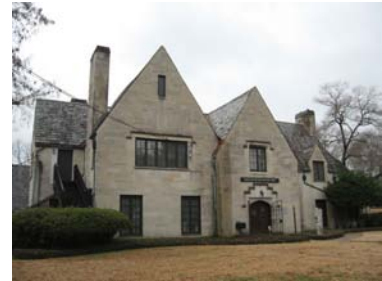
The Masur Museum's steeply-pitched gable roof is a signature of the Tudor Revival style. Altering this roof shape or form would adversely affect its expression of the style.
