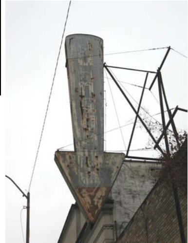
This mid-twentieth century, metal sign at 103-105 Catalpa Street incorporates neon lighting on its exterior, to outline lettering. This was a common style for the period.
