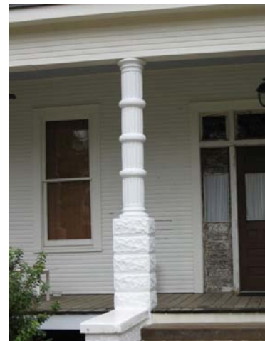
Original concrete porch column at 110 Hilton Avenue.
