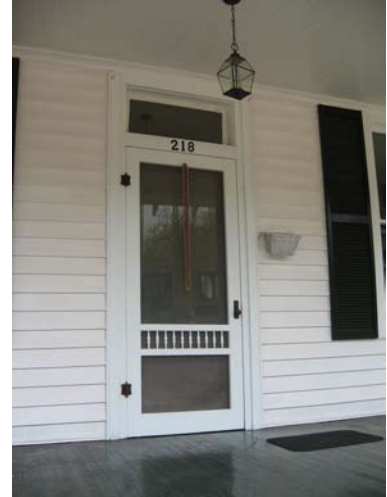
An appropriate screen door at 218 K Street does not conceal the original wood door behind it.
