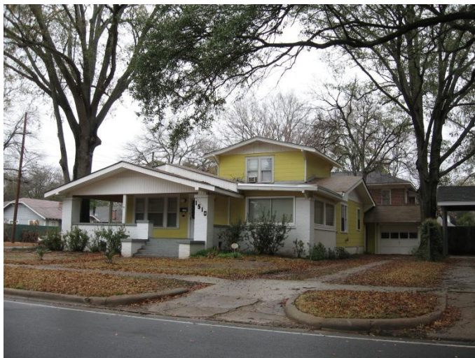
At 1510 3rd Street is an example of what is known as an Airplane Bungalow, which has a raised roof element and off-centered projecting bays with multiple gabled rooflines.
