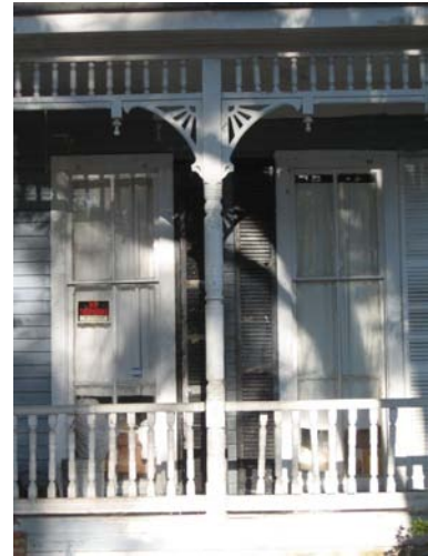
Porches like this one at 1205 St. John Street often have an abundance of wood elements, including milled posts, railing and balusters, and ornamental trim.
