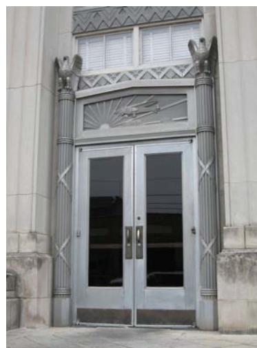
The distinctive entrance of the U.S. Post office enhances the character of the Art Deco building.
