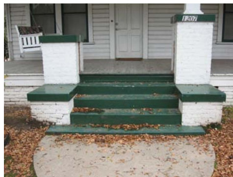
Original concrete steps at 1207 St. John Drive.
