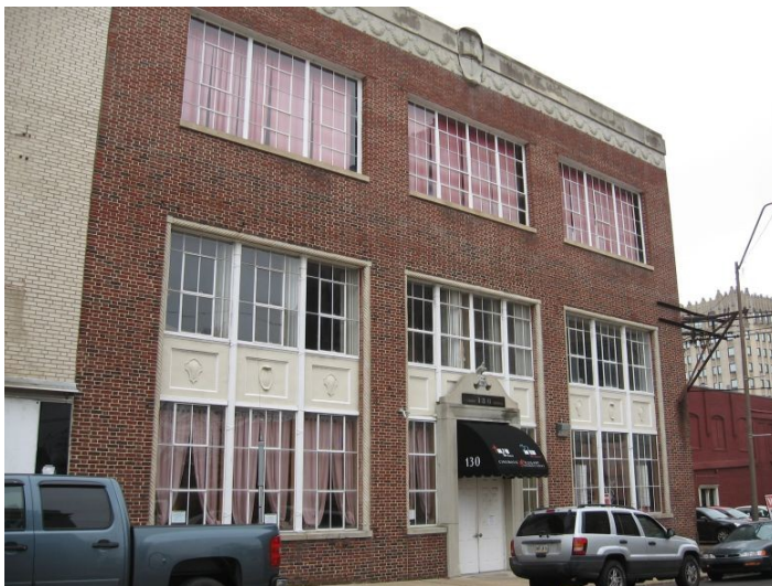
Pilasters divide the façade at 130 N. 2nd Street and present a balanced and symmetrical appearance.
