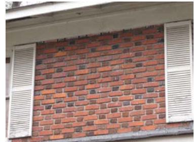
The Flemish bond brick exterior at 1010 N. 3rd Street adds an element of texture to the dwelling.
