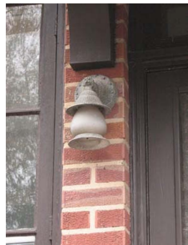
Original light fixture at 409 Auburn Avenue.
