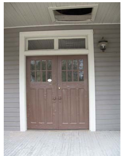
These eight-light, three-panel double doors should be maintained and preserved (1008 N. 3rd Street).
