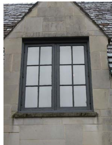
Original casement windows at 1400 S. Grand Street.
