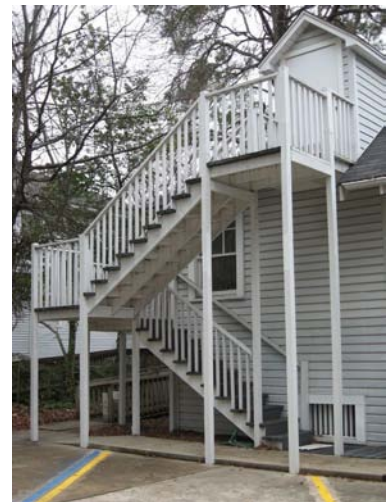
The stairs at 903 N. 2nd Street are located on the rear of the building.
