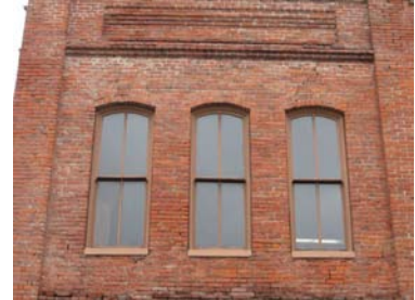
Original arched two-over-two wood sash windows at 101 N. Grand Street
