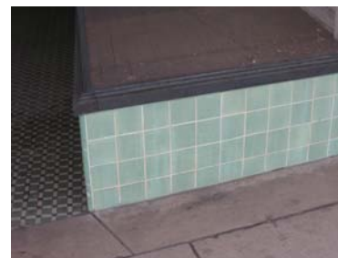
Tile bulkheads such as those at 406 Desiard Street (top) and 408 Desiard Street (bottom) are significant parts of storefronts from the early-to-mid-twentieth century.
