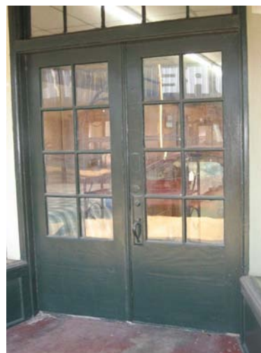
Original doors should be preserved and maintained such as at 504 Desiard Street (above) and 131 N. 2nd Street (below).
