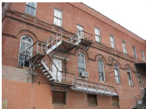
Fire escape at 125 St. John Street
