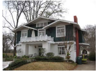
The contrasting colors between upper and lower stories of this Craftsman dwelling further differentiate the wood shingle siding on the top floor from the weatherboard siding on the lower floor (301 Park Avenue).
