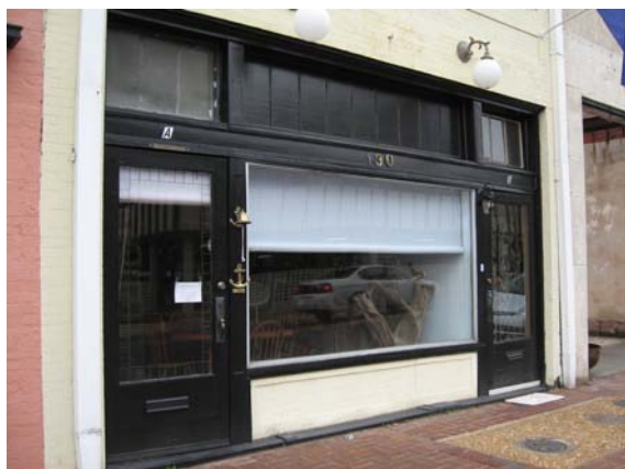
The original storefront at 130 S. Grand Street features single-light glass and wood doors, transoms, and a large central display window.
