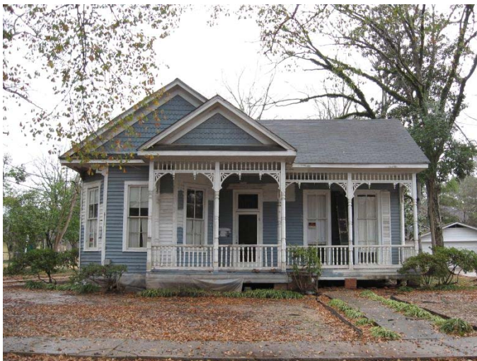
This gabled ell at 1205 St. John Street is a modest design with decorative spindles and post on its porch.
