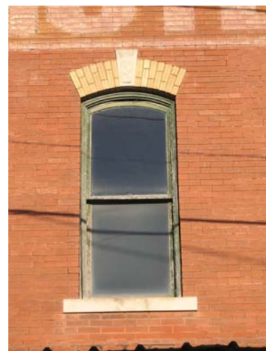
One-over-one arched window with segmental arch above at 500 Desiard Street
