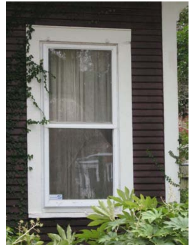
Storm windows like at 406 Auburn Avenue protect original windows and provide an insulating effect that make retaining historic windows more cost effective than replacing them.
