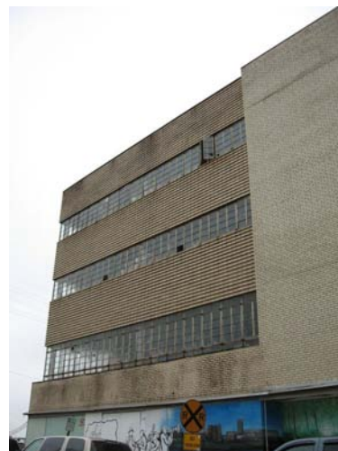
This 1950s building at 132 N. 2nd Street has an exterior of brick and steel casement windows.
