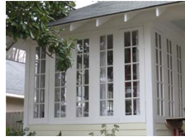
The original casement windows of this sunroom help define the historic character of the dwelling (400 McKinley Street).
